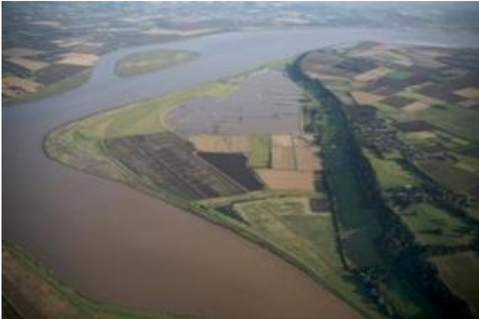
Figure 2.7b The Alkborough Flats Managed Realignment site after the breach of the flood defences (WildlifeExtra, 2008).
