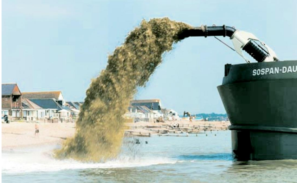
Figure F7 An offshore rainbow dredger replenishing Pevensey Bay in East Sussex (Website 22)
